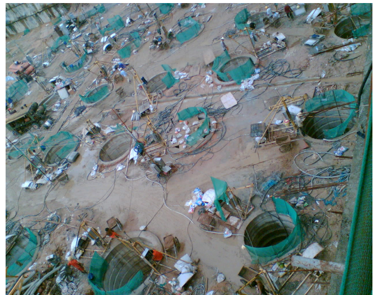
FIGURE 4a- Tower Pile Construction
