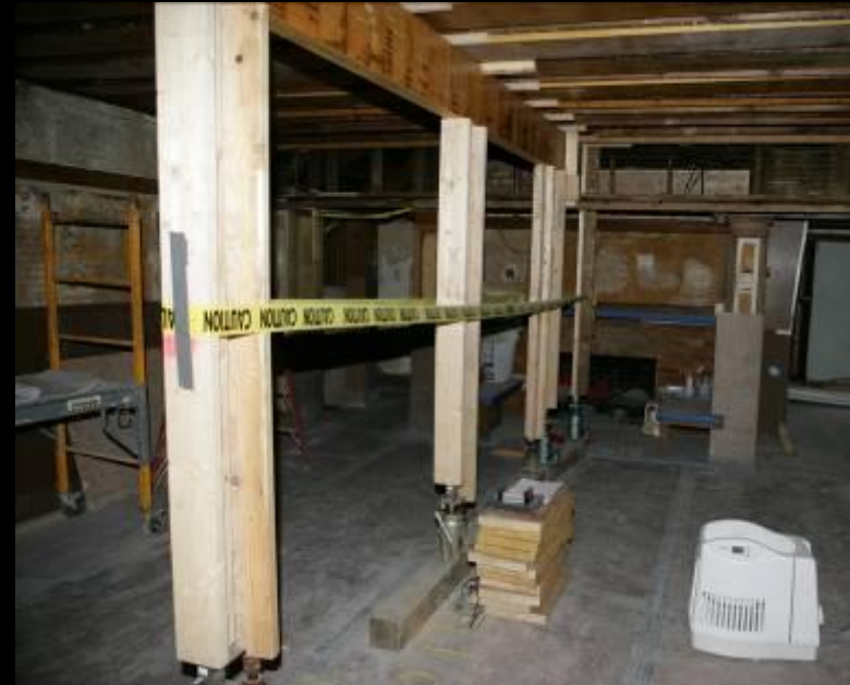
Straighten Walls and Level Floors
