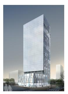
Thornton Tomasetti completed schematic design for a 34-story office tower and six-story above ground podium for the Block A1 Spec Tower in the master-planned Songdo International Business District, in Incheon, South Korea. In addition, we completed design development for the basement and the tower foundation. Since the structure sits on reclaimed soil, the two-meter-thick mat foundation sits on two-meter diameter piles.
