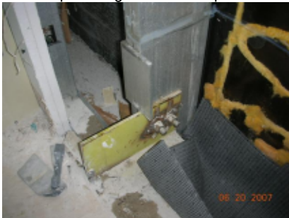
Repaired mullion connection
