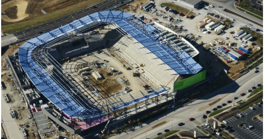
Courtesy Turner Construction
