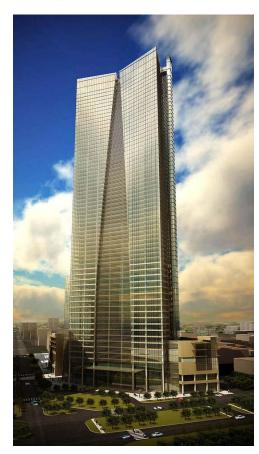
At 270 meters, the Lotte Center Hanoi will be the tallest building in Vietnam upon completion. Thornton Tomasetti was retained by the owner to provide structural peer review and value engineering consulting services for the 253,395-gross-square-meter, mixed-use tower. The 65-story tower accommodates office, residential and hotel spaces above grade, and parking and mechanical spaces on five below grade levels.
